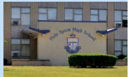
Holy Spirit High School in Absecon, New Jersey, has a more efficient and less costly heat system thanks to new high-efficiency gas heat system.
