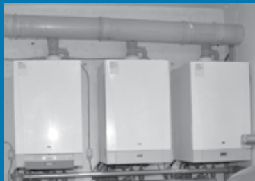
Central Baxi high efficiency boiler plant
